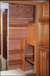
Cedar-lined closet with built in shoe rack.
